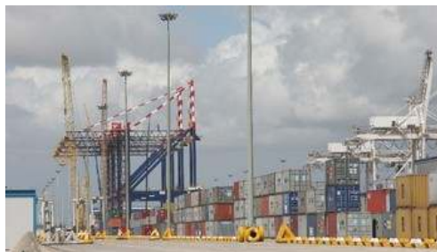
LEFT: New container cranes taking shape in Cape Town
